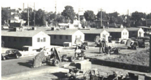
U.S. Army ordinance depot, Westlake Avenue North and North Valley Street, Seattle, 1943
