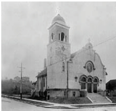
The first St. Anne Church, completed in 1908, stood on the corner of Lee Street and 2nd Ave. W. Its stucco walls did not last long in the damp Northwest climate.
